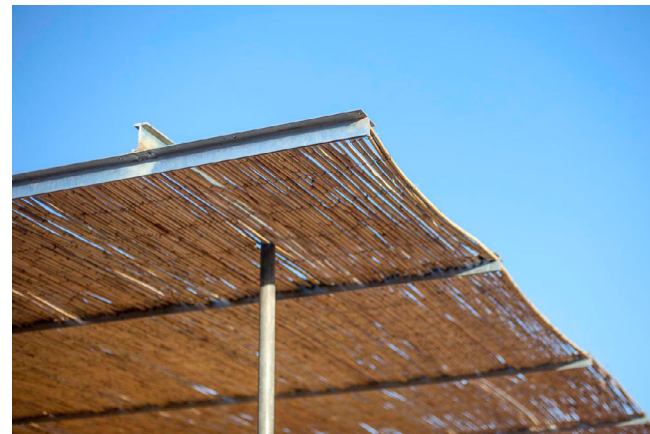
Natural reed pergola. Typical of the area
